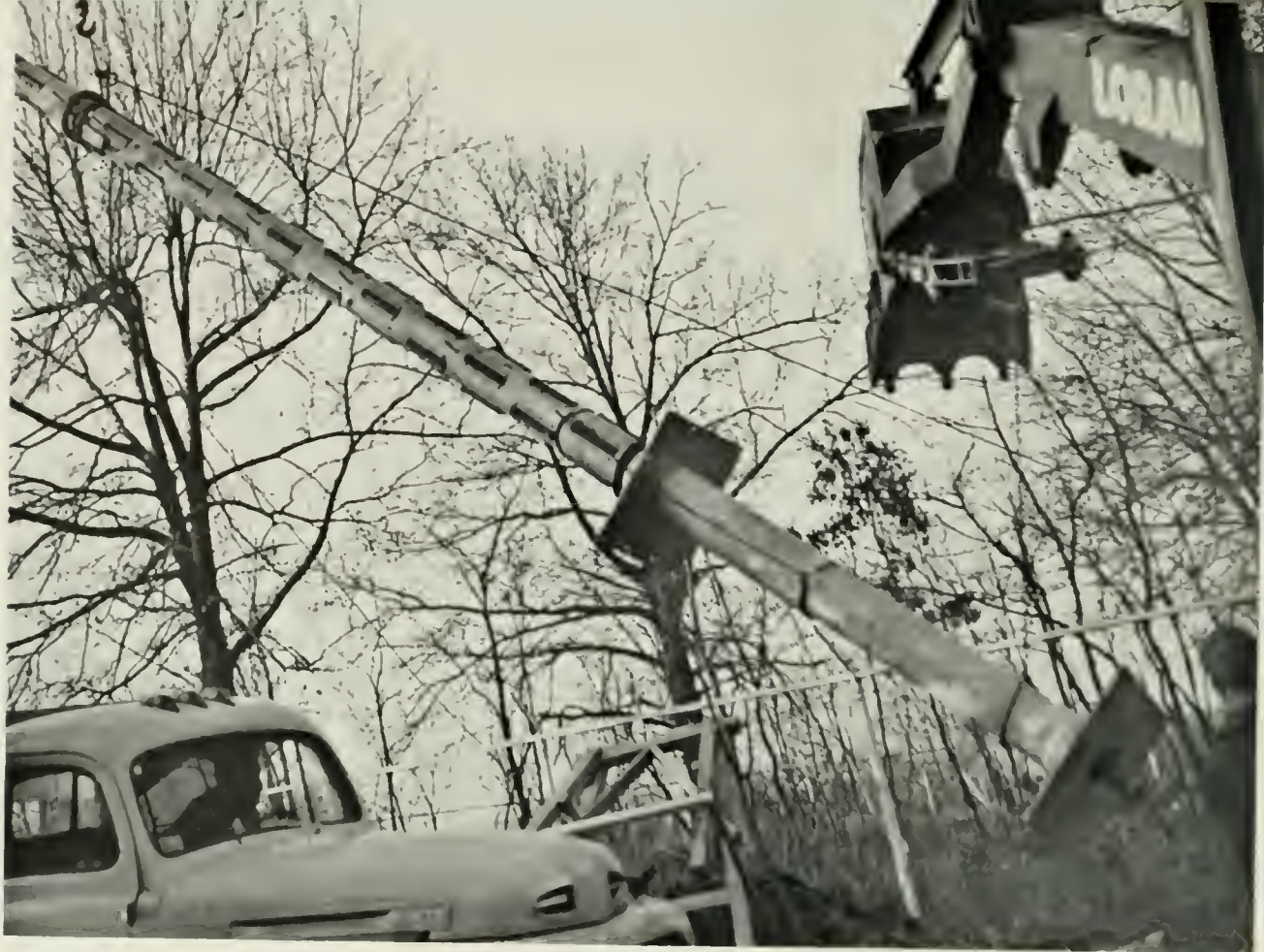
WORKMEN HOIST THE 40-FOOT UHF ANTENNA INTO PLACE AT NBC'S NEW EXPERIMENTAL TELEVISION STATION NEAR BRIDGEPORT, CONN.
